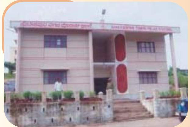
Town Police Station, Sakleshpur
