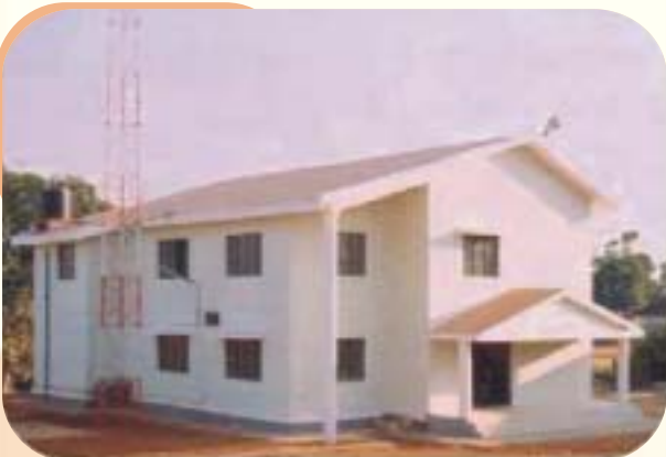
Rural Police Station, Hosanagara
