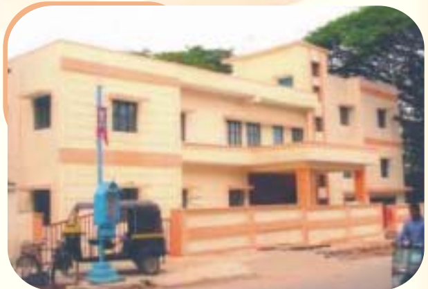
Shivajinagar Police Station
