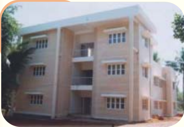
West Town Police Station & Women Police Station, Pandeshwar, Mangalore
