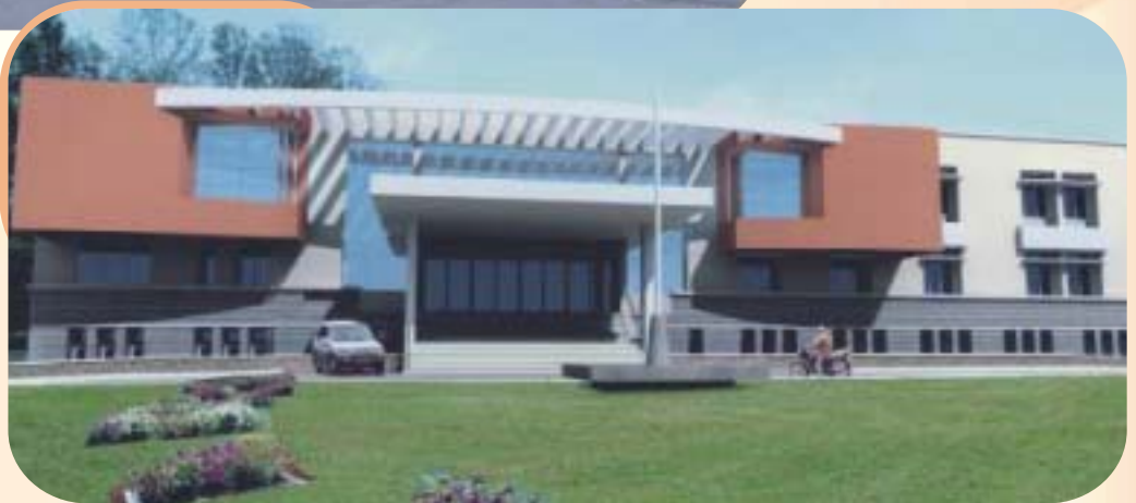
Multi-functional IGP / SP office complex at Belgaum under construction
