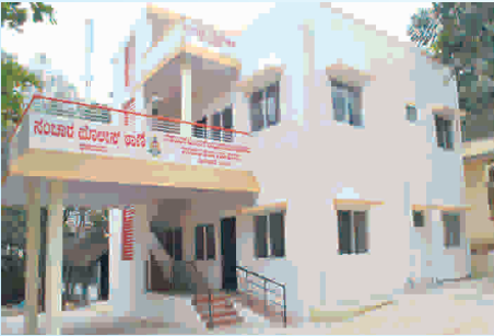
Traffic Police Station, Dharwad
