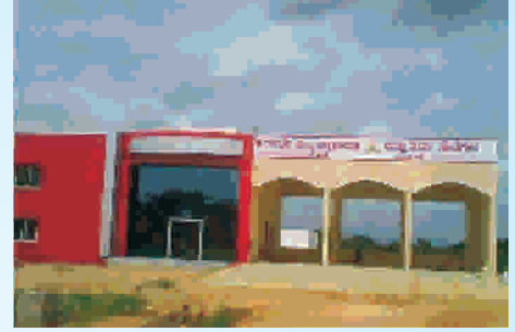
3 Bay Fire Station, Malavalli, Mandya
