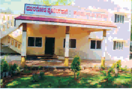
Police Station, Muragod, Belgaum
