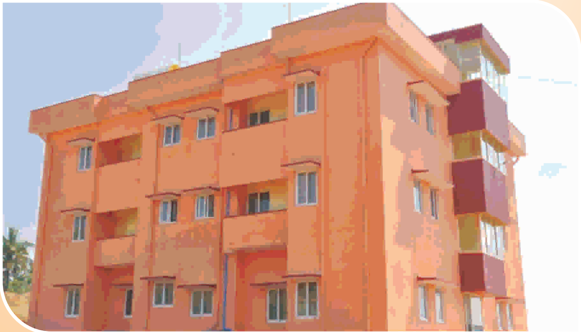
12 PC Quarters for Coastal Security Police, Shivalli, Udupi
