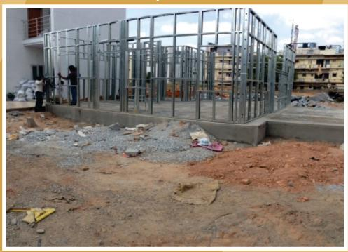
Composite construction – Light gauge steel skeleton
