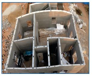
Fig.11 – G. F. Wall structure ready Foam concreting top view.
