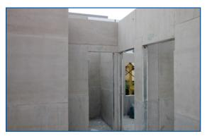
Fig.20 – Inside view of cement fiber board Fixing on 1st floor
