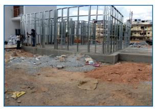
Fig.5 - Erection of LGS Wall Structure
