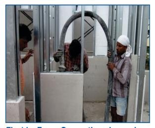
Fig.14 – Foam Concreting closer view.
