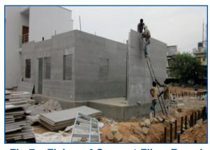
Fig.7 - Fixing of Cement Fiber Board
