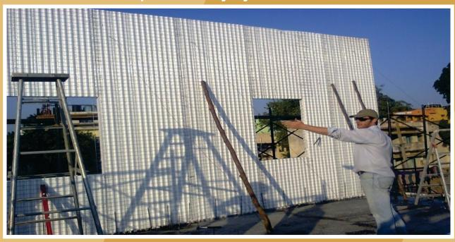
Baupanel technology Expanded Polystyrene panels in position
