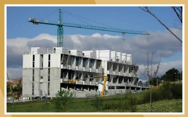
Picture 2. 8 storey Baupanel building under construction
