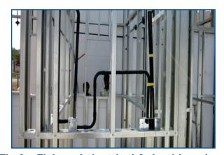
Fig.8 – Fixing of electrical &plumbing pipes
