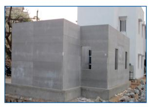
Fig.9 – G.F.Wall structure ready for Foam concreting rear view.
