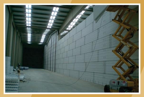
Picture 4. 12 m height partition wall in a warehouse
