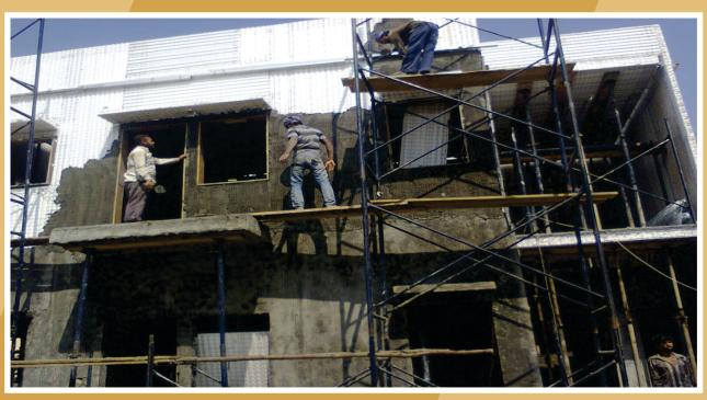
Application of micro concrete to polystyrene wall panels under progress
