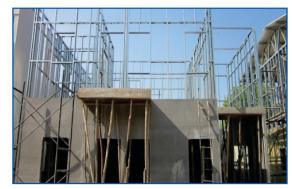
Fig.17 – Erection of LGS wall structure for first floor.
