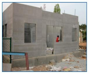
Fig.10 – G. F. Wall structure ready for for Foam concreting front view.
