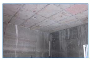
Fig.21 – G.F.roof slab after removing the centering.
