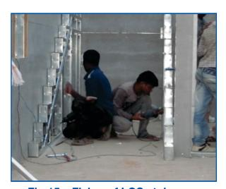
Fig.15 – Fixing of LGS staircase.
