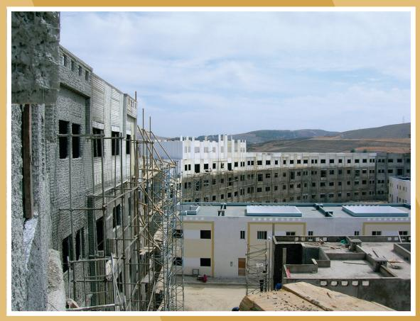
Picture 3. Huge housing development using Baupanel system.
