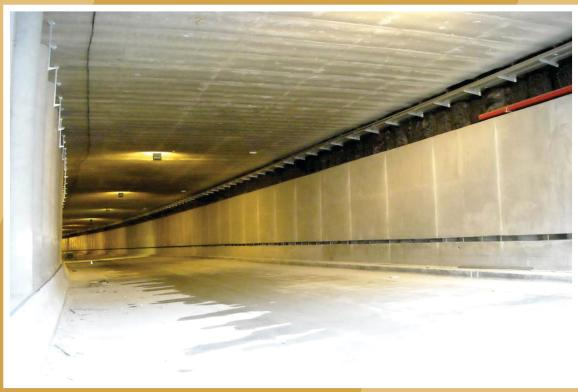
Picture 5. Sheeting of a pile wall in 2 km length tunnel
