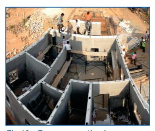
Fig.12 - Foam concreting in progress.
