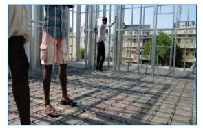
Fig.16 – Steel reinforcement for G.F.roof slab
