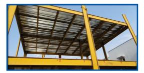
Roof Slab deck sheeting with concrete.
