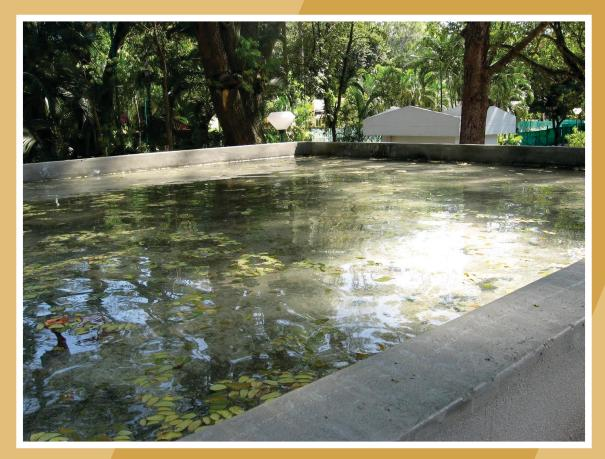
Ponding test by storing water on roof slab in progress
